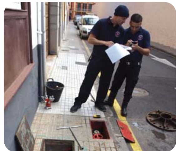
Review of the hydrant network
